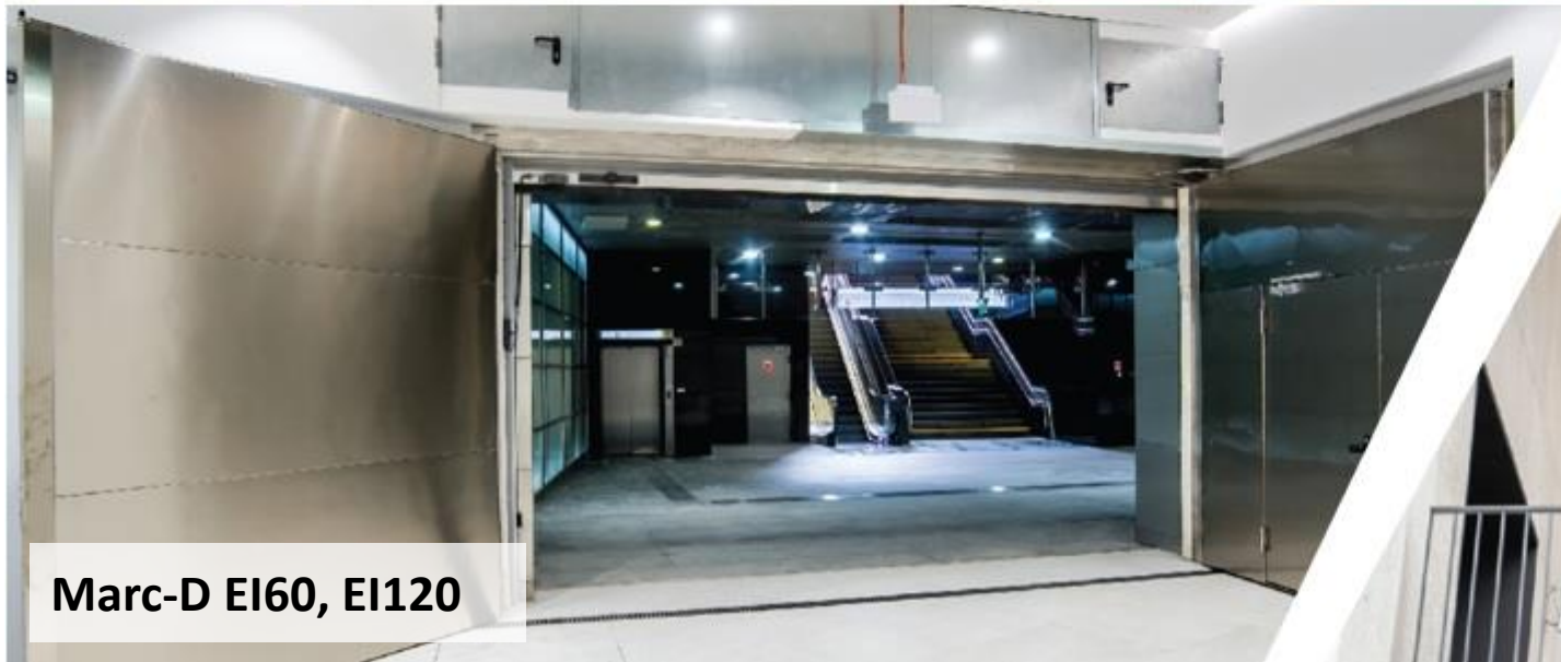
Handling system fire closures EI30 EI60 EI120
